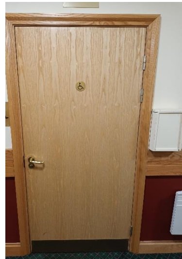
Brandling House 2 nd Floor
